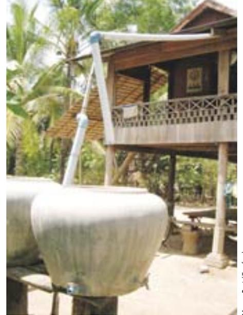
Very low cost rooftop rainwater harvesting using corrugated iron roof, hard plastic pipes and ferro-cement jars for storage at a home in Cambodia.
