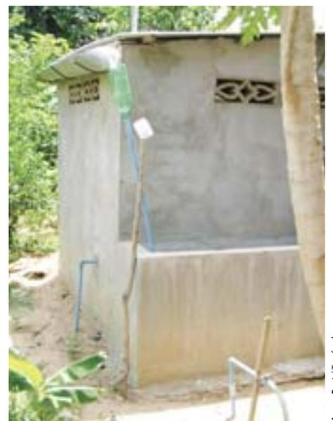
Rainwater harvesting off the roof of a latrine in Cambodia, using an old soft drink bottle, hard plastic pipe, corrugated iron and a brick storage tank. This concept is especially useful as it provides water for hand washing right at the door of the latrine.
