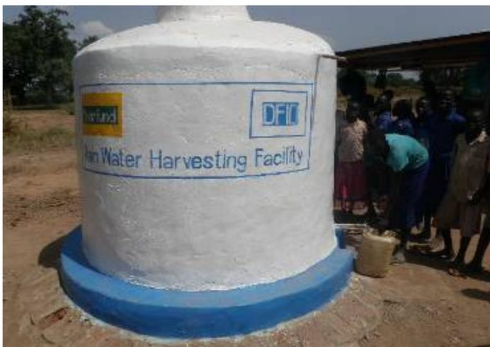
**Photo:** A ferrocement tank constructed at a school in Omdurman
