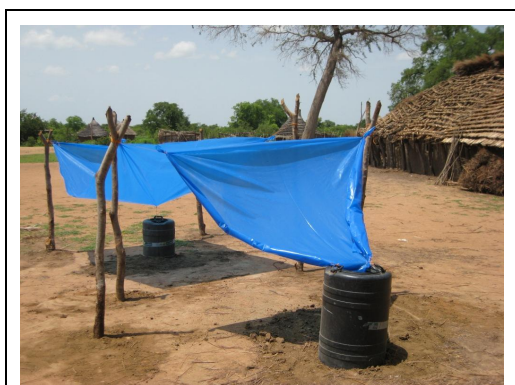
Photograph 1. Example of Plastic Sheet Rainwater Harvesting Systems
